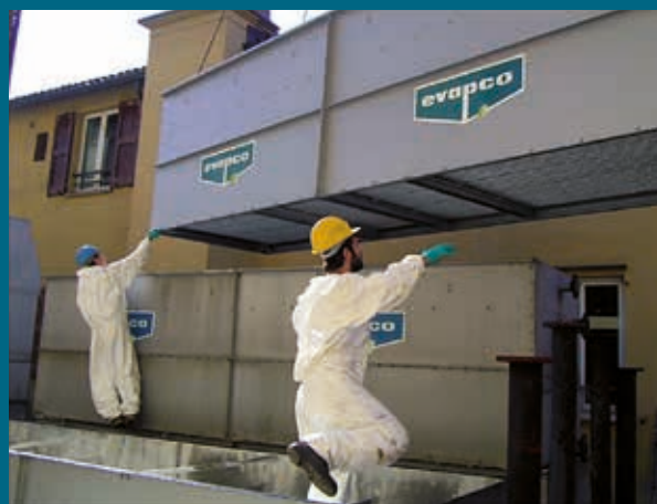
Complete section replacement
