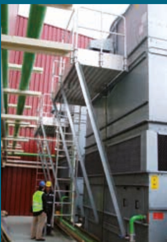
Ladder & Platform Installation
